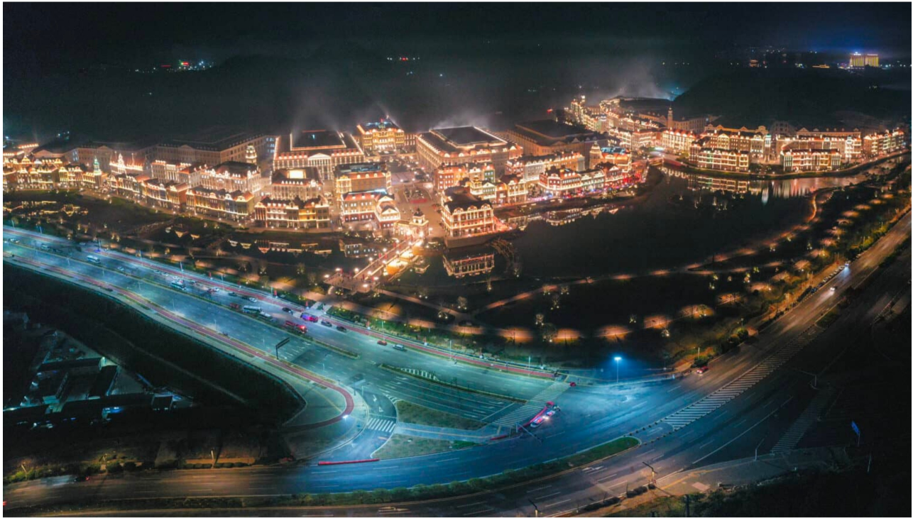
An aerial view of Huawei's data center in Gui'an New Area during its opening ceremony on December 20, 2021 in Gui'an, Guizhou, China. Credit: VCG via Getty Images
