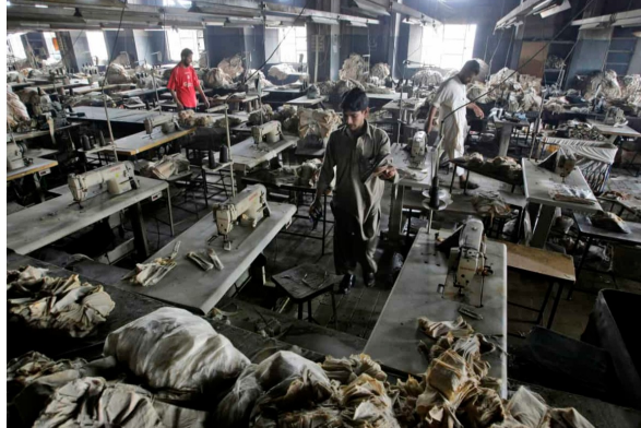
Pakistani men check a burnt garment factory in Karachi, Pakistan, 13th September 2012, after a fire broke out two days before. The previous month, August 2012, the factory was issued an SA8000 certificate by RINA SpA. Credit: Fareed Khan via AP Photo
