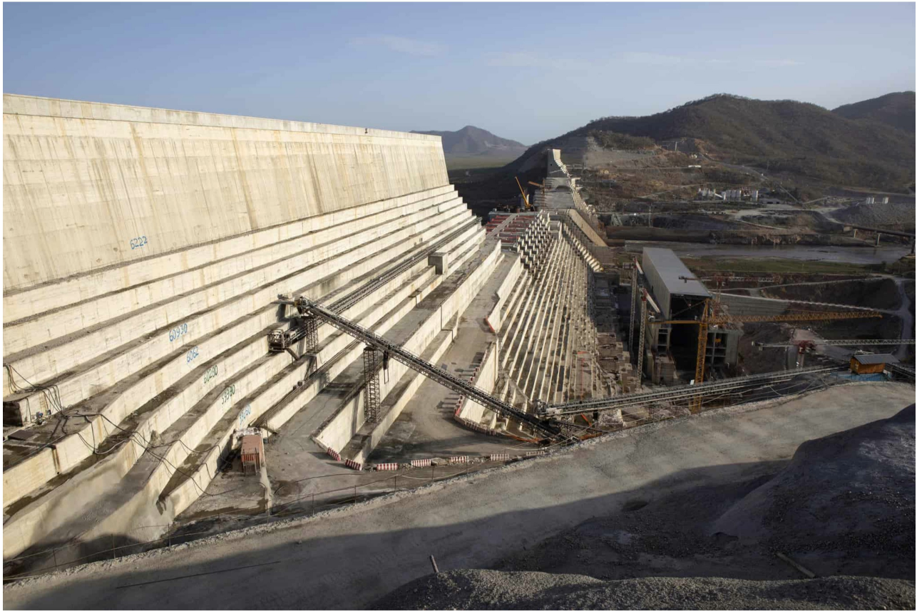
Construction progress on the Grand Ethiopian Renaissance Dam, partially financed by China, a massive project that Ethiopian leaders promised would make the country energy independent. But the dam has stoked tensions with Ethiopia's neighbors. Credit: Bloomberg/ Getty Images
